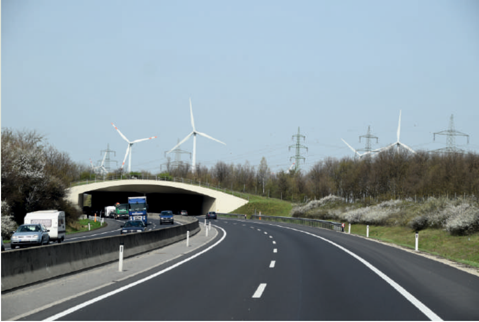
ph. 77 | Mitigating of cumulative impact of different infrastructures on landscape is of a great challenge. Budapest-Vienna Motorway, Austria (© L. Georgiadis)
