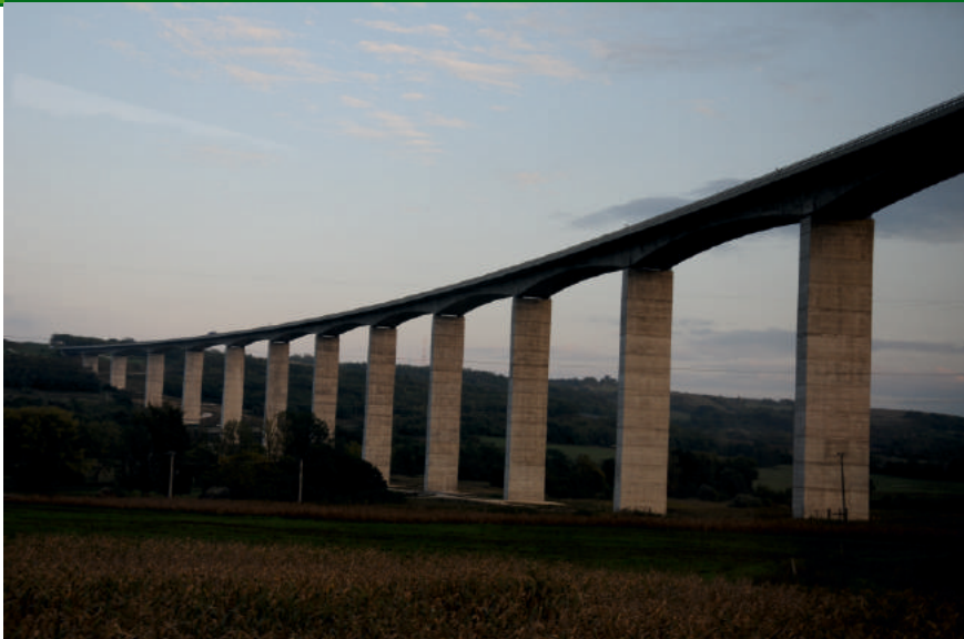
ph. 49 | Long Viaduct in Hungary. Field trip during IENE 2010 Conference (© L. Georgiadis)
