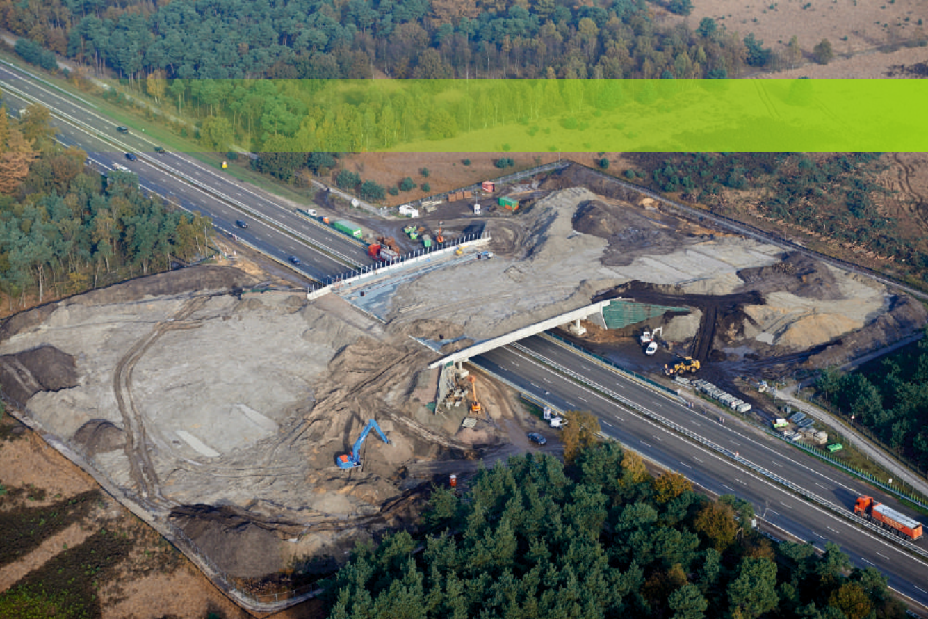
ph. 55 | Ecoduct Groote Heide over highway A2 south of the city of Eindhoven, the Netherlands (© Jacob Van Den Borne)
