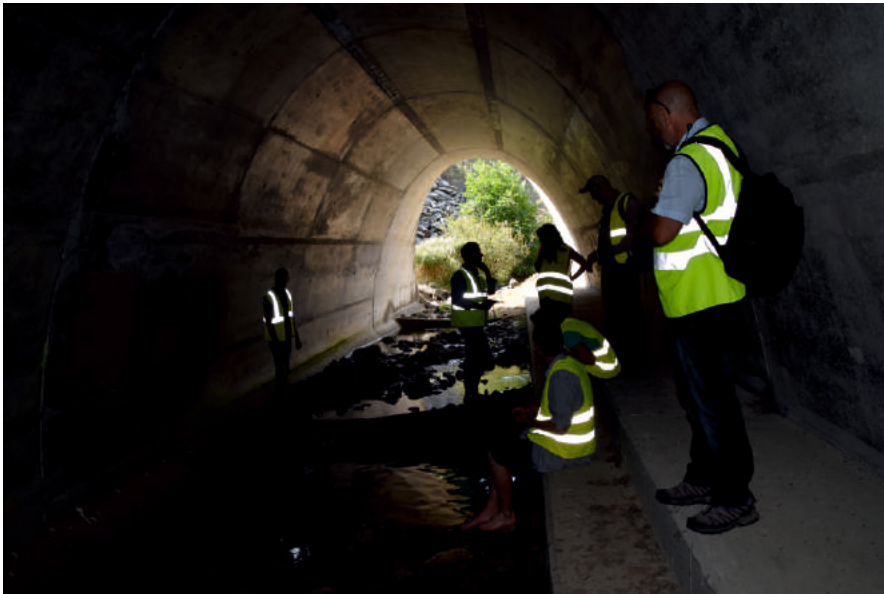
ph. 54 | Inside of an underpass water crossing in France during the Field visit in IENE 2016 International Conference in Lyon (© L. Georgiadis)
