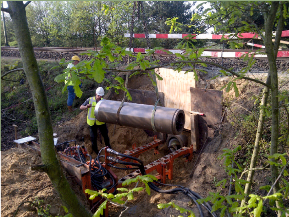
ph. 61 | Ecological engineering on defragmentation of railway fragmented habitat, Netherlands (© ProRail)
