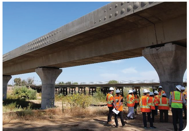
Illustration 3 - Overpasses and underpasses may be adapted (a) to facilitate wildlife use providing vegetated strips and screens to reduce noise and visual disturbance from traffic circulating under the structure.
