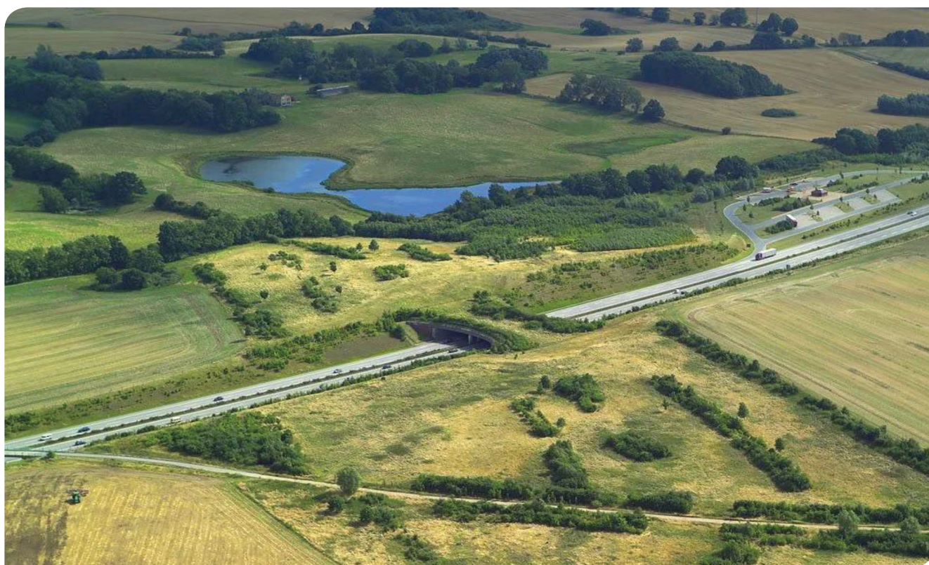
Illustration 2 - Ecoduct near Barnekow across the A20 in northern Germany The bridge reconnects grassland and shrub habitats that have been recreated on both sides of the motorway © DEGES, René Legrand, https://www.deges.de/projekte/projekt/vde-10-a20/
