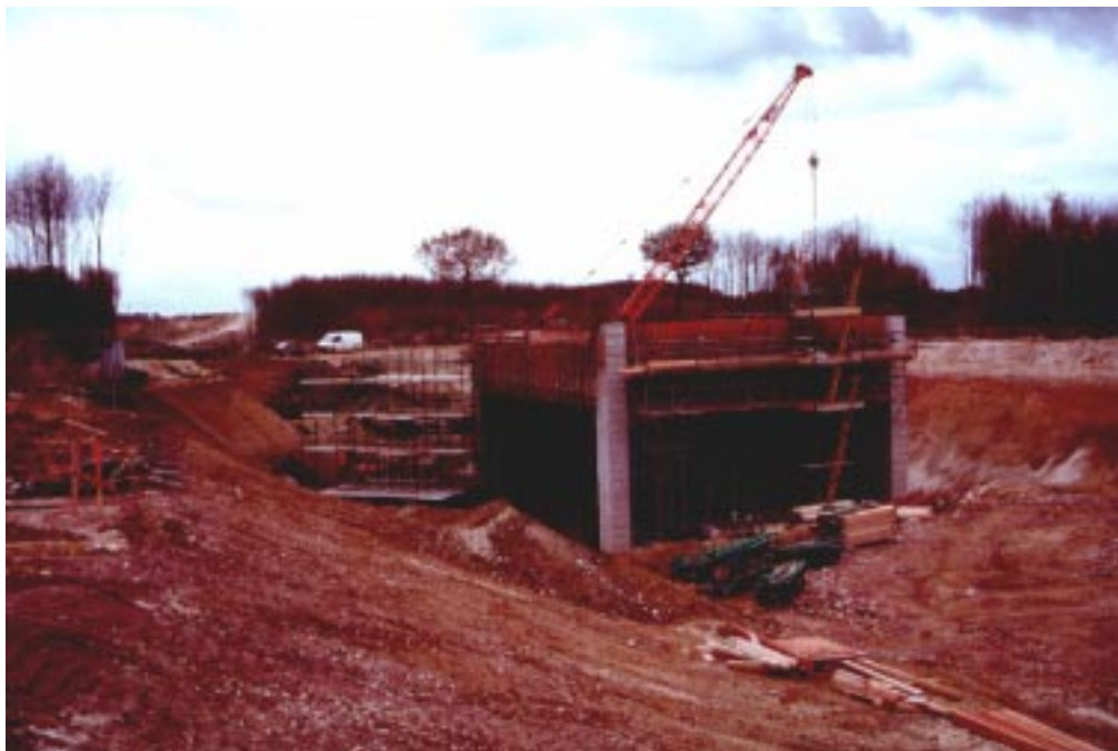
Figure 7.17 : Construction of Land Bridges over CTRL route (November 1999) (RLE)
