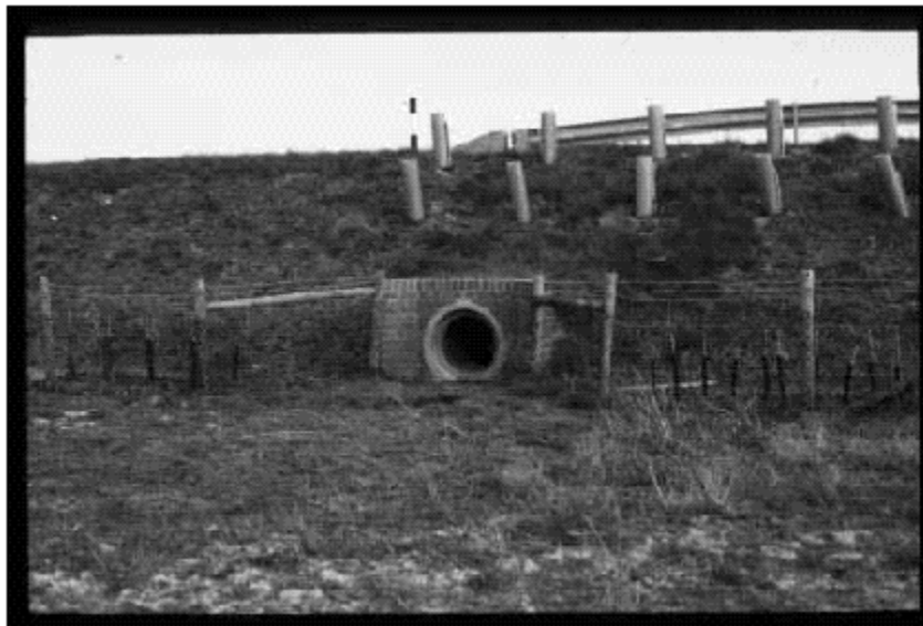
Figure 7.3: Ideal underpass design for badgers and otters using fencing to guide animals to the entrance
