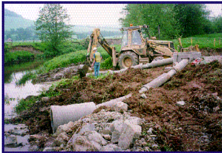
Figure 7.7: Installing an artificial otter holt
