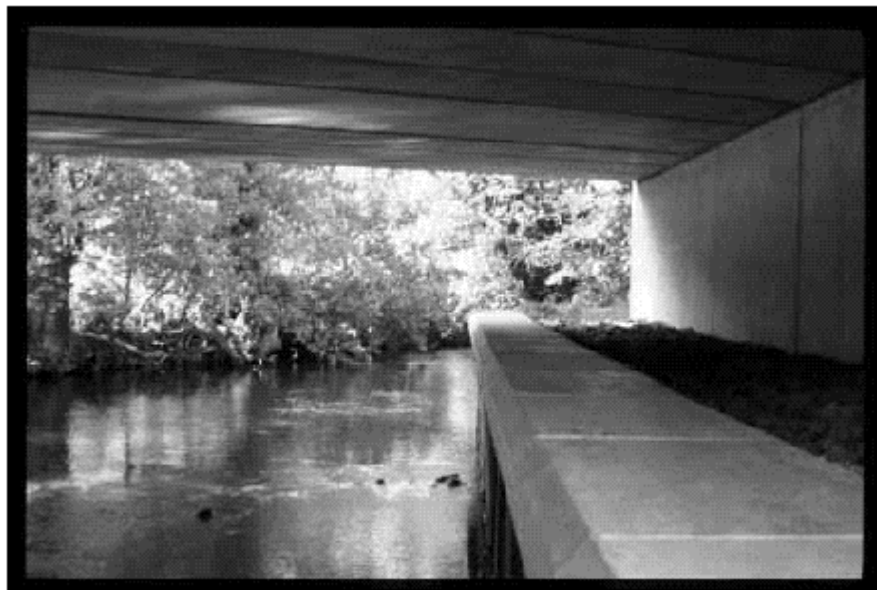
Figure 7.15. Hole Bridge, Bovey Tracey, Devon. A ledge was incorporated into the bridge design during construction.
