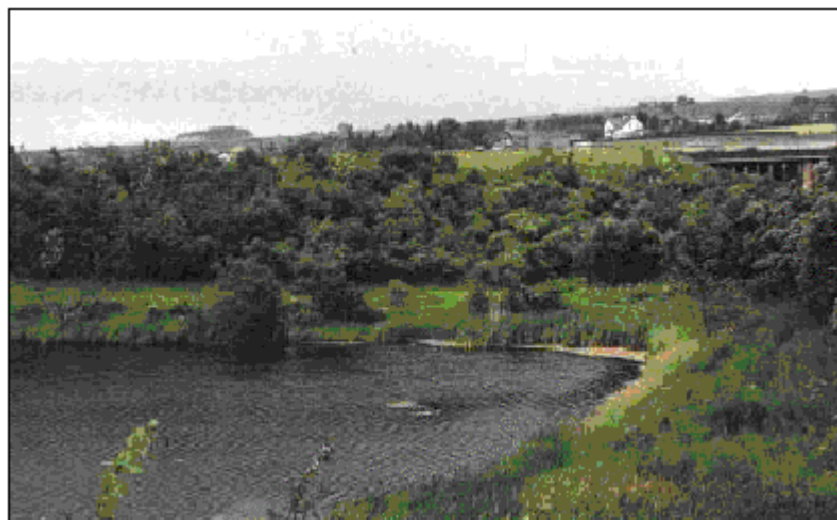
Figure 7.10: Good practice in balancing pond design M6, Lancashire. Shallow edges have created the right conditions for reed beds and wet grasses
