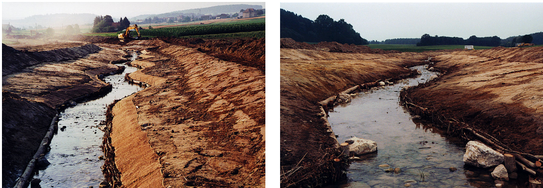
Figure 7.11 - Widened river bed of the Arignon in the canton of Fribourg, which in addition to its ecological functions will provide flood protection.
