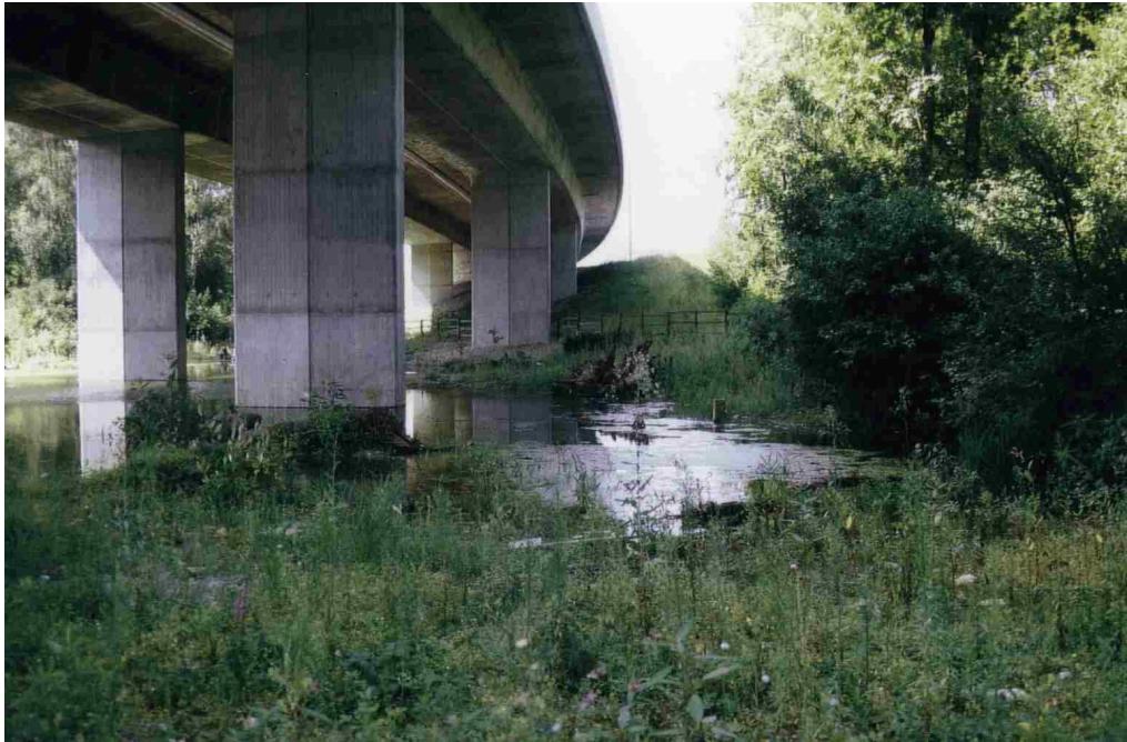
Figure 7.3 - The bridge for the A3 in the Schinznach region, constructed instead of the planned embankment. (Source: Baudepartement des Kantons Aargau)
