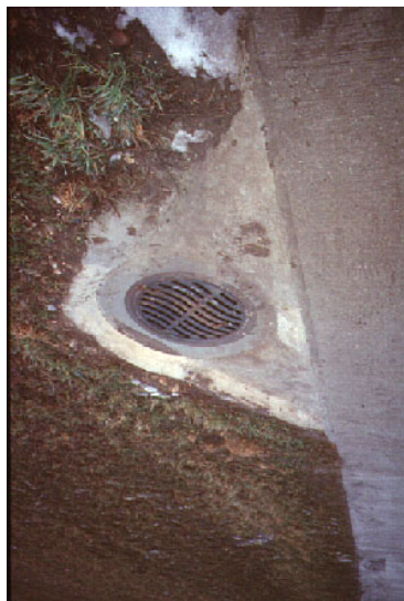
Drainage via shoulder or with drain without kerbstone (photo: KARCH)
