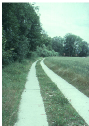
An example of a farm lane with load bearing strips (photo: A. Ducommun)
