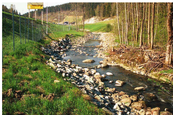
Figure 7.4. Photograph of the new river bed and culvert of constructed for Årungselsva as it ran close to a stretch of the E6 Akershus, Norway, being upgraded to dual carriageway. Under construction and after. (Photos: B. Iuell)
